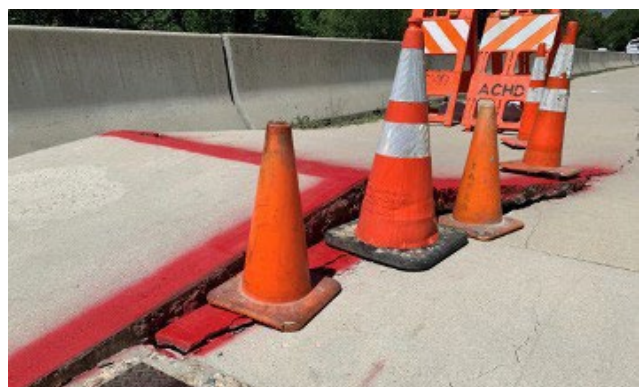
Figure 1. Heat-related pavement buckle on Veterans Memorial Parkway in Boise. Photo: Ada County Highway District.
